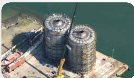
Two SO 2 converters for a nickel mine in Madagascar. Built on the quayside of ND Engineering's Bayhead workshop, these 500 t modular plants were shipped as completed units.
