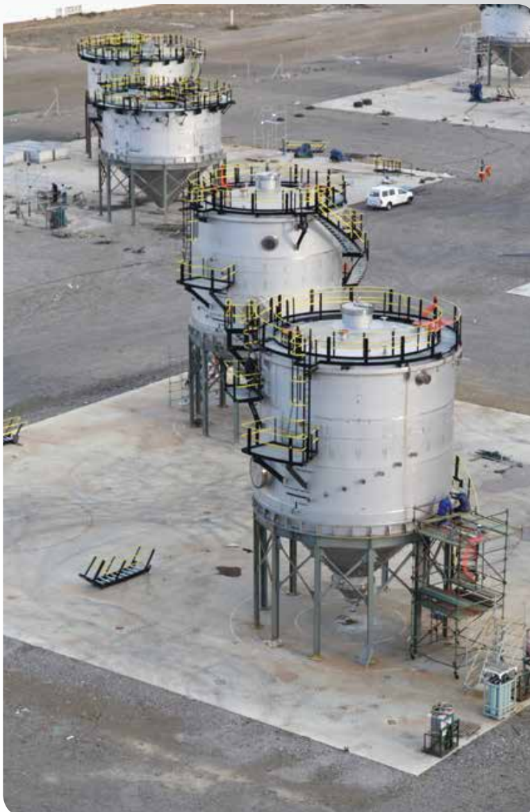
Complex tar separator vessels for a Sasol processing plant in Secunda. These vessels involved duplex materials from 8,0 mm to 50 mm and, according to Green, “the most comprehensive welding procedures we have ever seen”.
