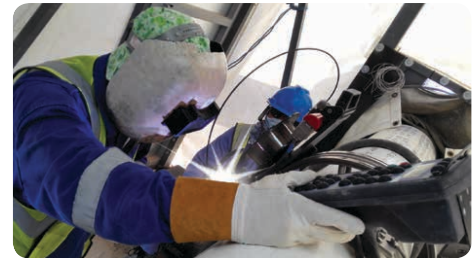
Figure 4: Orbital welding equipment is suitable for use on-site for pipe laying, in harsh environmental conditions.
