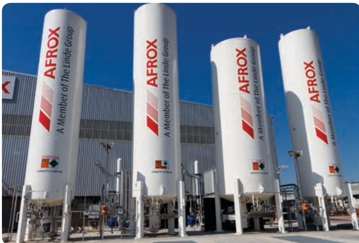
Four cryogenic storage tanks dominate the Riverhorse Valley skyline. The plant takes delivery of liquid CO 2 , Nitrogen, Oxygen as well as Argon from Pretoria.
