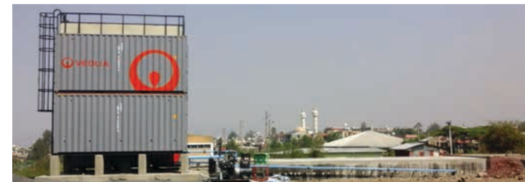
Above: Veolia supplied a 100 m 3 /day hybrid modular sewage treatment plant (STP™) for Ethiopian Airlines' cargo terminal at Addis Ababa International Airport in under 16 weeks (ex-works).
