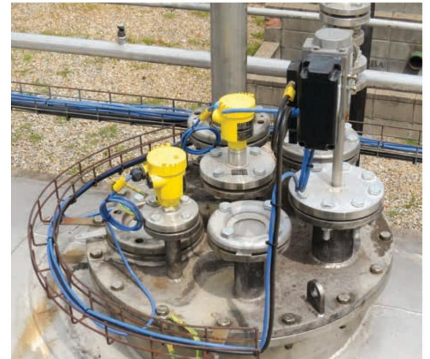
The narrow radar beam of the VEGAPULS 64 sensor allows it to be installed where metal elements exist.
