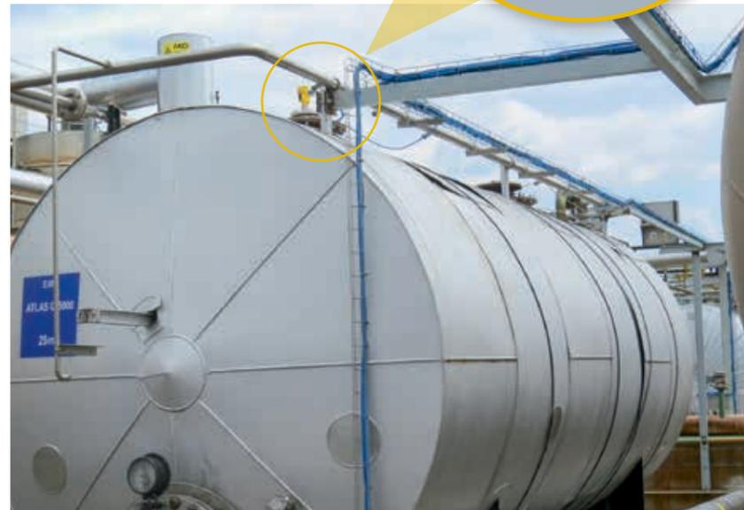
On tanks for storing raw materials, the VEGAPULS 64 allows non-contact filling level measurement down to the bottom of the tank despite internal installations such as heating coils.
