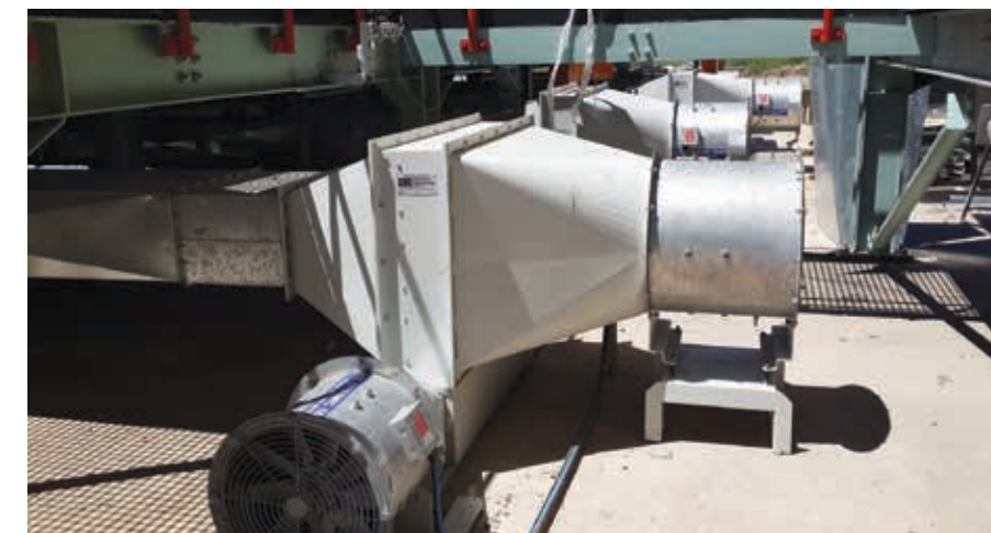
When using spin filters for back channel cooling, ambient air from outside the control centre is channelled through a VSD, over the heat sink of the device, then vented out from the MCC.
