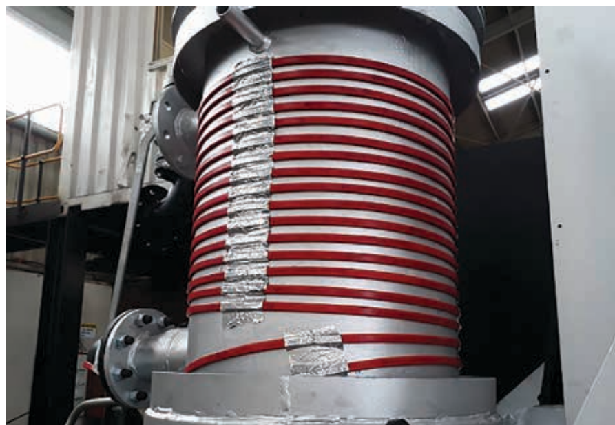
EHT lowers the viscosity of many processes as it acts as a compensating heat source to maintain or raise the heat in pipes, tanks, surfaces and other vessels.
