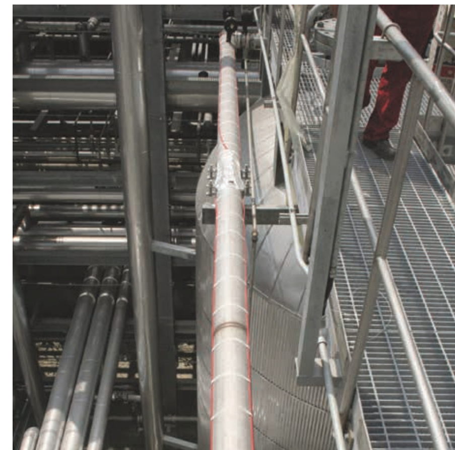
EHT enables manufacturers to keep products at an optimal temperature, lowering viscosity and ensuring that it is easier to transport fluids around the plant during the colder months.
