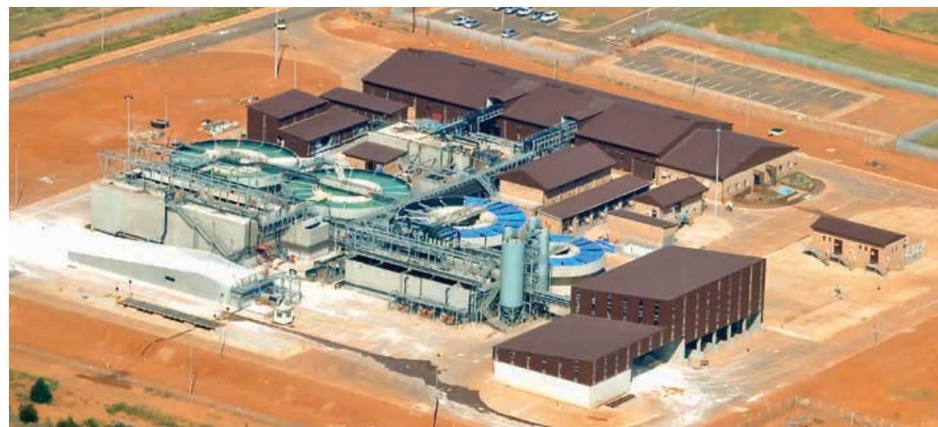
The Middelburg Water Reclamation Project (MRWP), developed by Aveng Water on an EPCM contract, is a 20 Ml/d mine-impacted water (MIW) treatment plant that produces 7.3-million m 3 of potable water per annum. Photo: Aveng Water.
