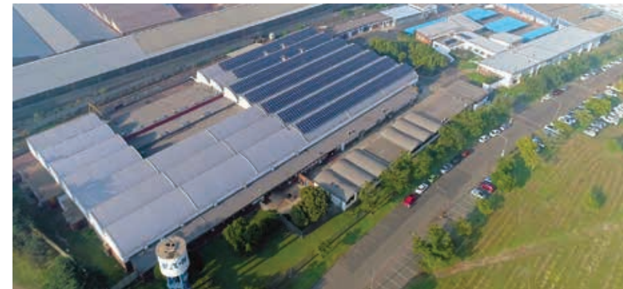
A 200 kW p rooftop solar photovoltaic system has been installed on the roof of Eaton's Wadeville facility.
