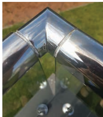
Examples of sub-standard stainless steel balustrade installation in KwaZulu-Natal.
