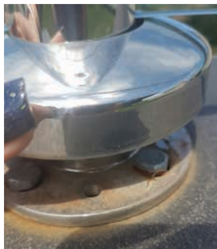
Examples of sub-standard stainless steel balustrade installation in KwaZulu-Natal.
