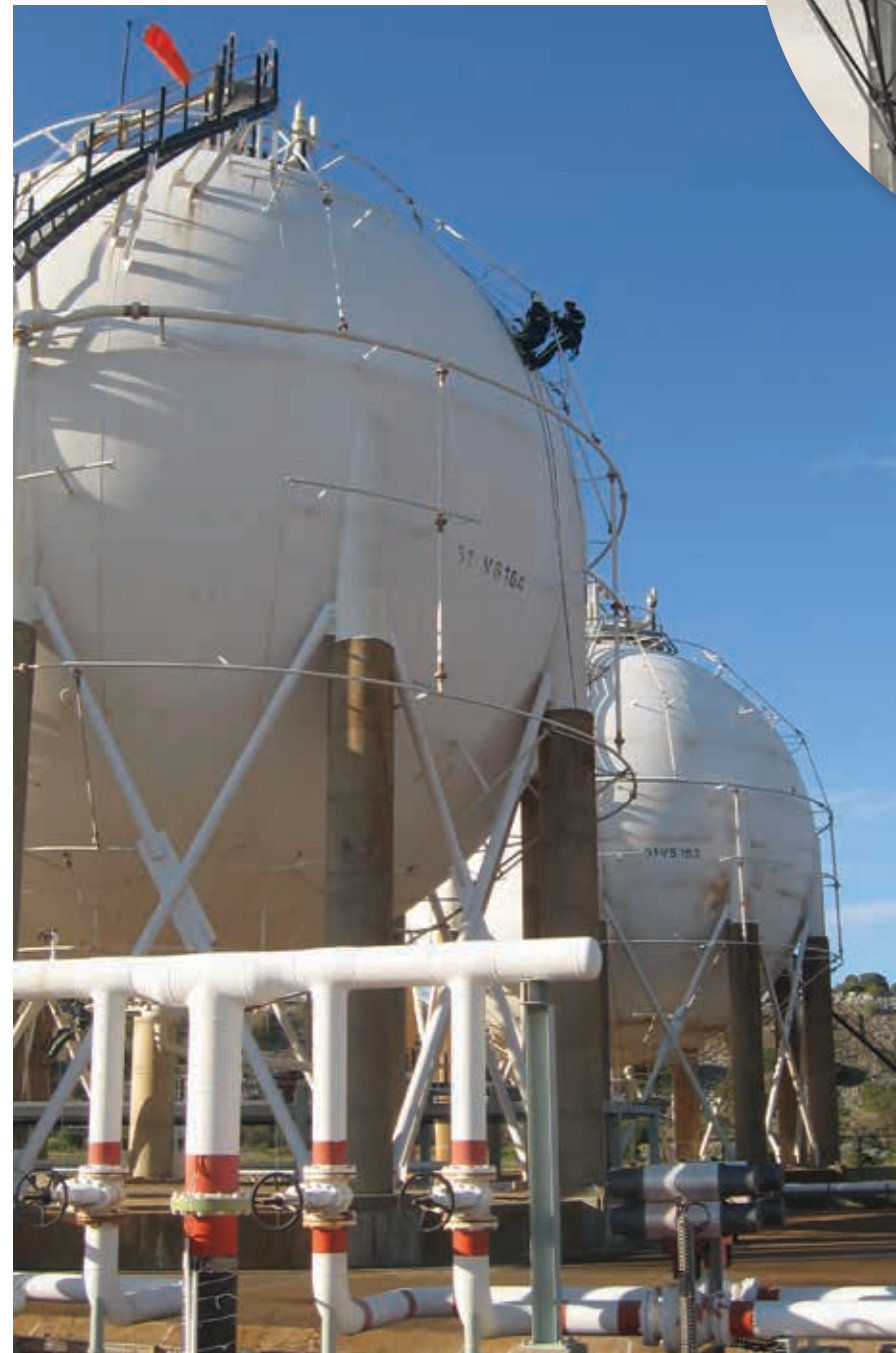
Technicians used rope access to reach the 14 m high roof and carried out UT wall-thickness measurement on select steel members.
